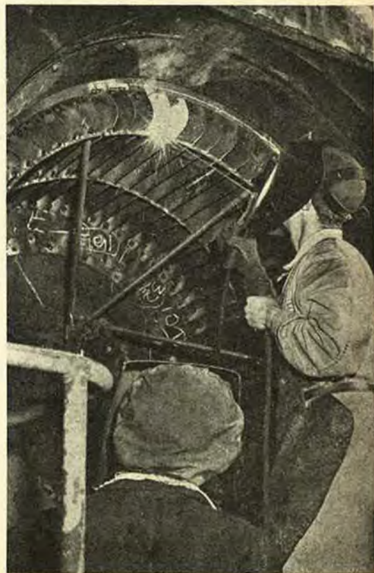
Welders Ron Geisman and Ray Hough repair the blades of an induced draft fan at Richmond.
