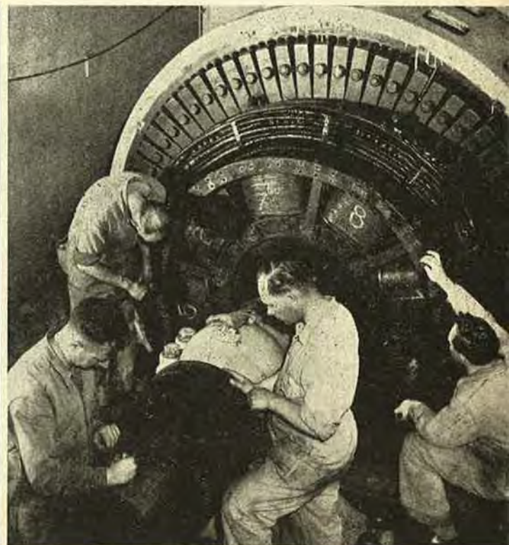
Left: Colin Sinclair is brazing rotor blades to the lacing wire of one of Newport's high pressure rotors. Right: Overhauling a synchronous condenser is comparatively rare maintenance operation.
